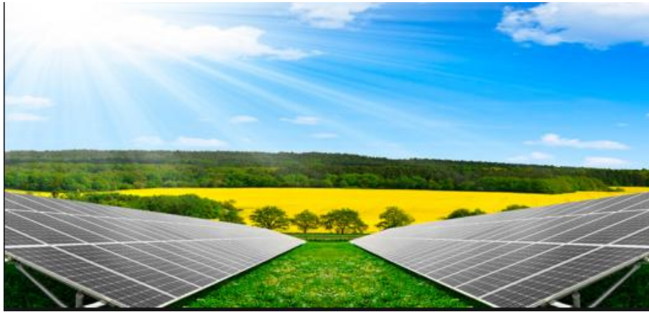
Fig.1 Solar PV system
